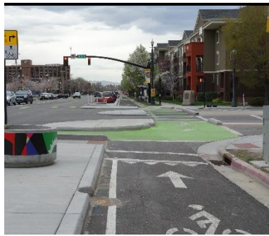
Type II – With Protected Bike Lane Intersection
