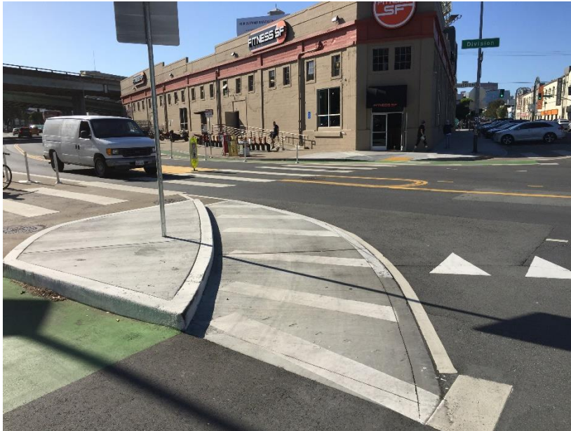
Figure 3-3 Example of Truck Apron (San Francisco, CA)
