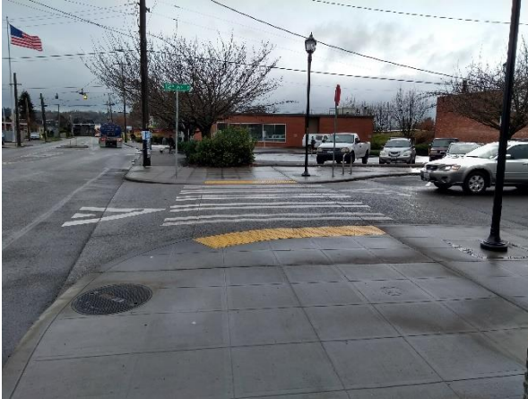
Figure 6-1 Example Side Street Seattle, WA
