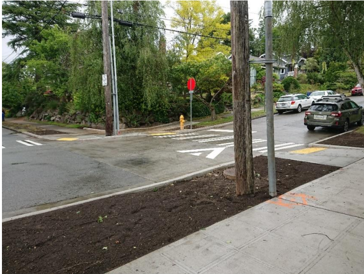
Figure 6-7 Raised Crosswalk on a Steep Street (Seattle, WA)
