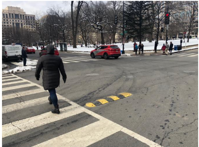
Mountable Hardened Centerline (Credit: Tom Bertulis)
