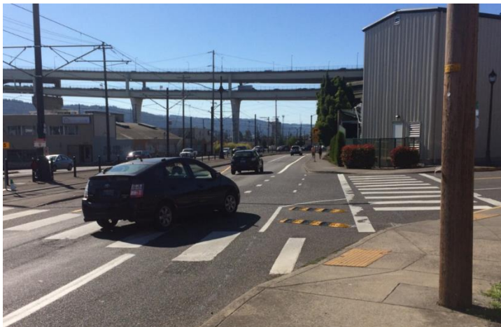
Figure 3-5 Example of a Turn Wedge (Portland, OR)
