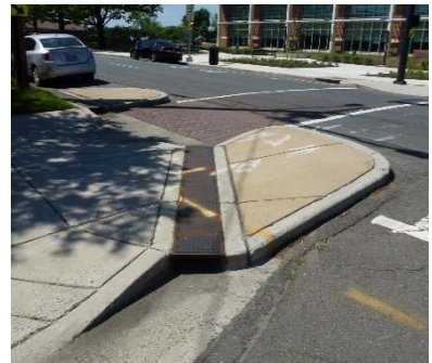
Type II – With Sidewalk Culverts
