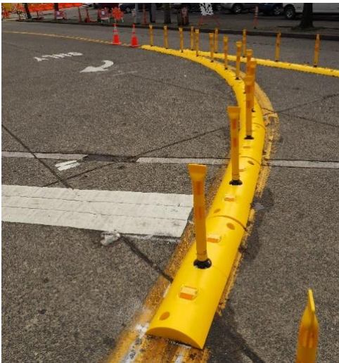
Flexible Delineator Hardened Centerline
