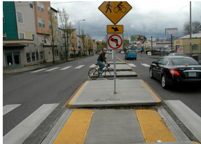
Intersection Crossing Island
