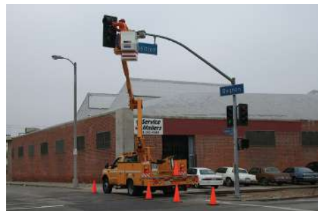
TRAFFIC SIGNAL REPAIR CREW
