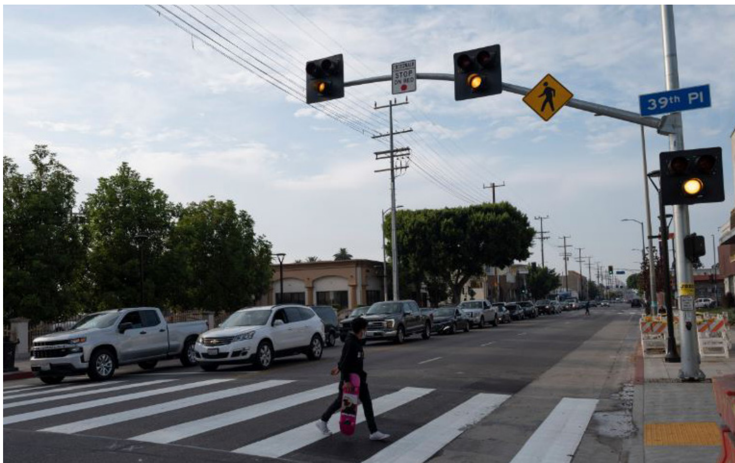
Newly Installed High Intensity Activated CrossWalk (HAWK) at Western Ave and 39th Pl
