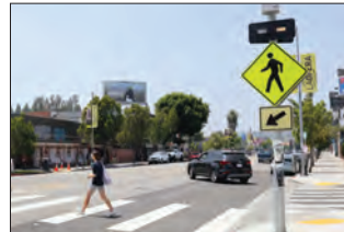
Pedestrian Flashing Beacons
