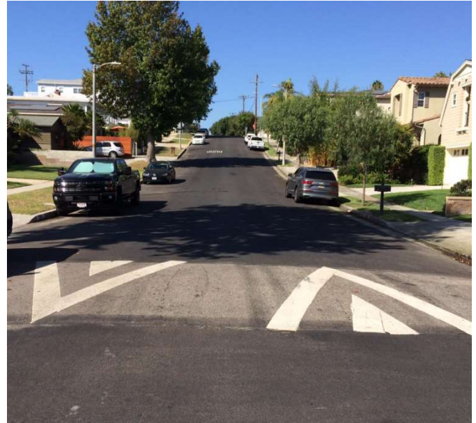
Image for Note 8: This speed hump is located on a section of the block where the grade is less than 7% but as far up the hill as possible
