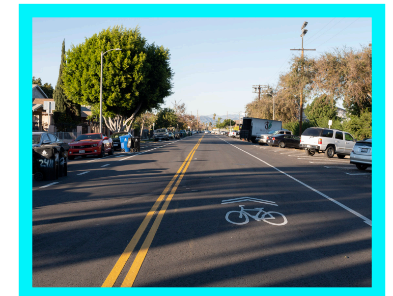
Marked with signs and painted sharrows but no dedicated road space for bikes
