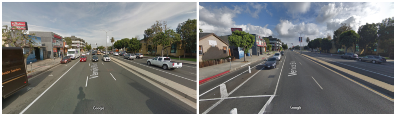
Figure 2 - 6 to 4 lane reconfiguration with parking protected bike lane on Venice Boulevard, Los Angeles
