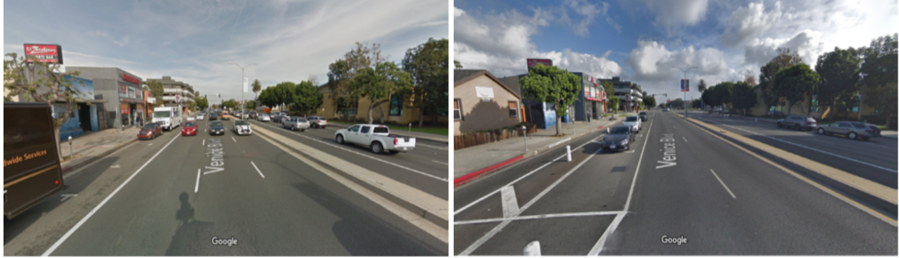
Figure 2 - 6 to 4 lane reconfiguration with parking protected bike lane on Venice Boulevard, Los Angeles
